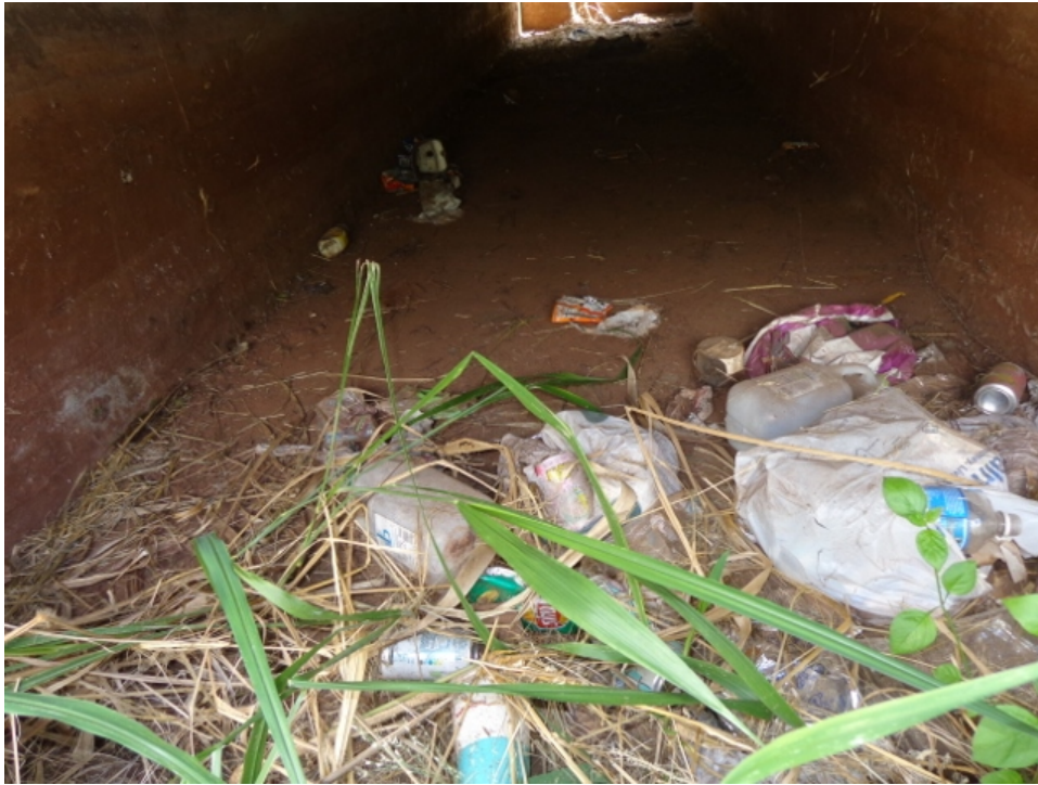
Photo 23: View of culvert invert
