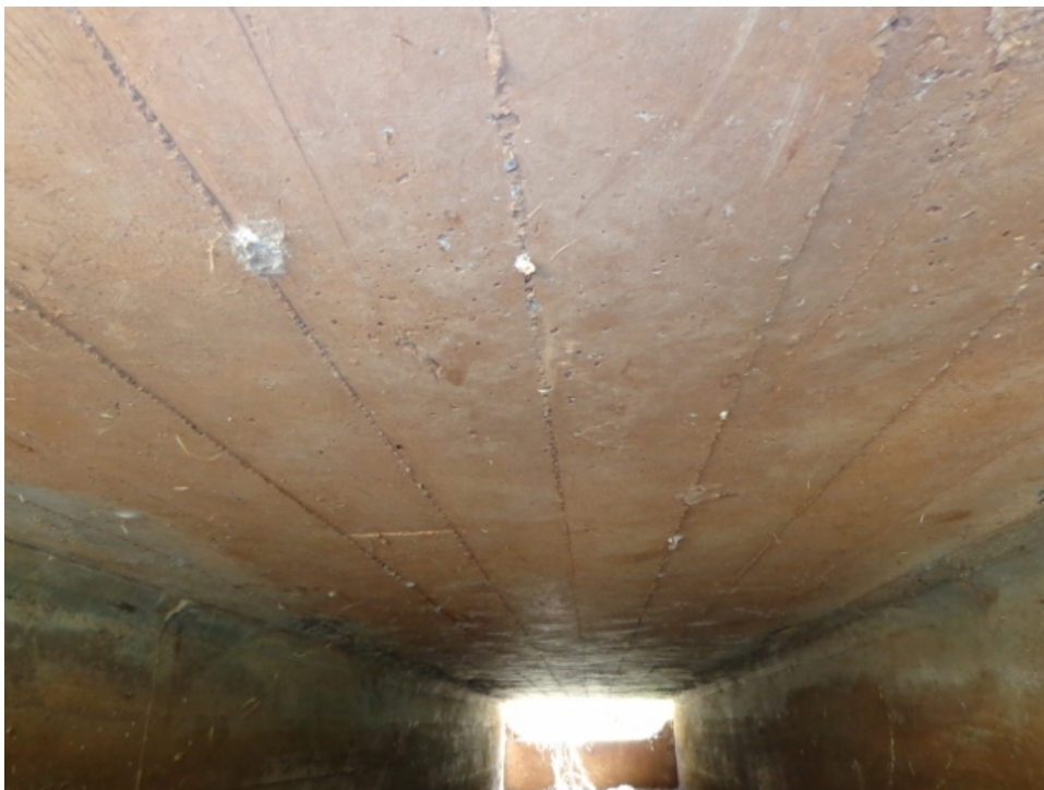
Photo 16: View of culvert soffit
