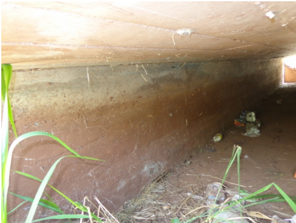
Photo 20: View of east culvert wall
