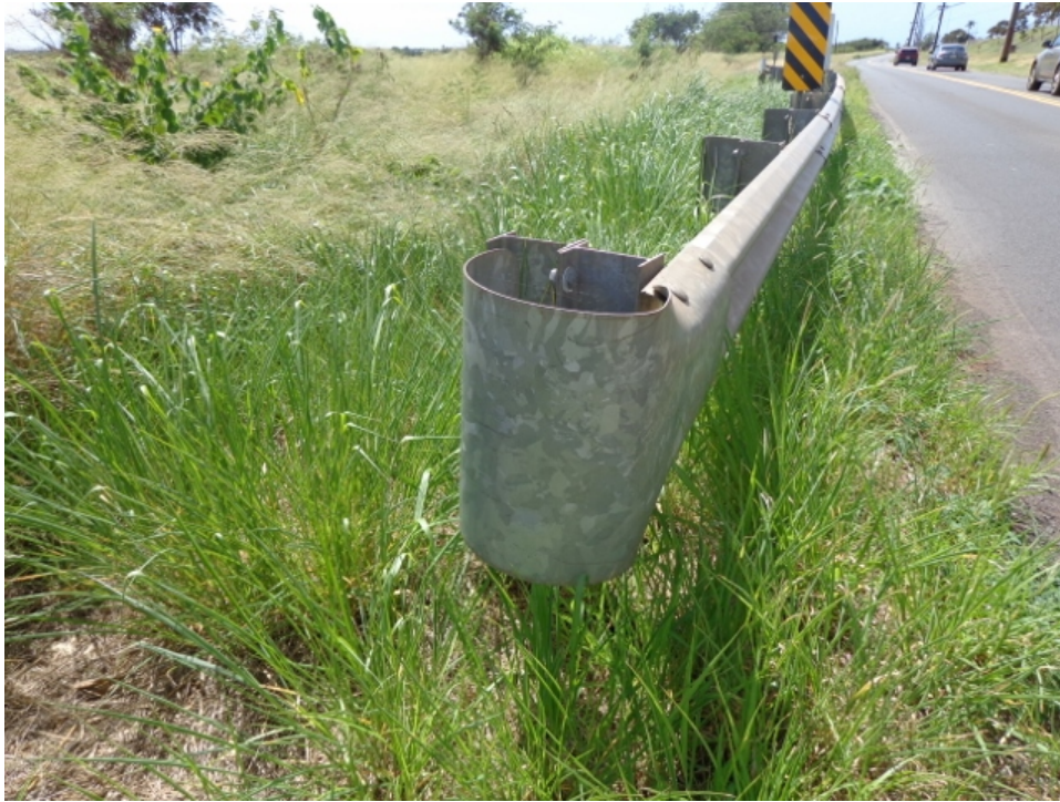
Photo 3: Downstream east approach guardrail end
