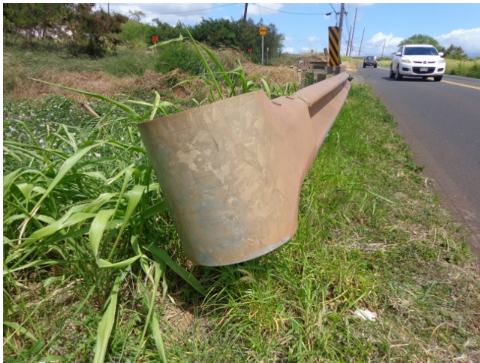
Photo 6: Upstream west approach guardrail end
