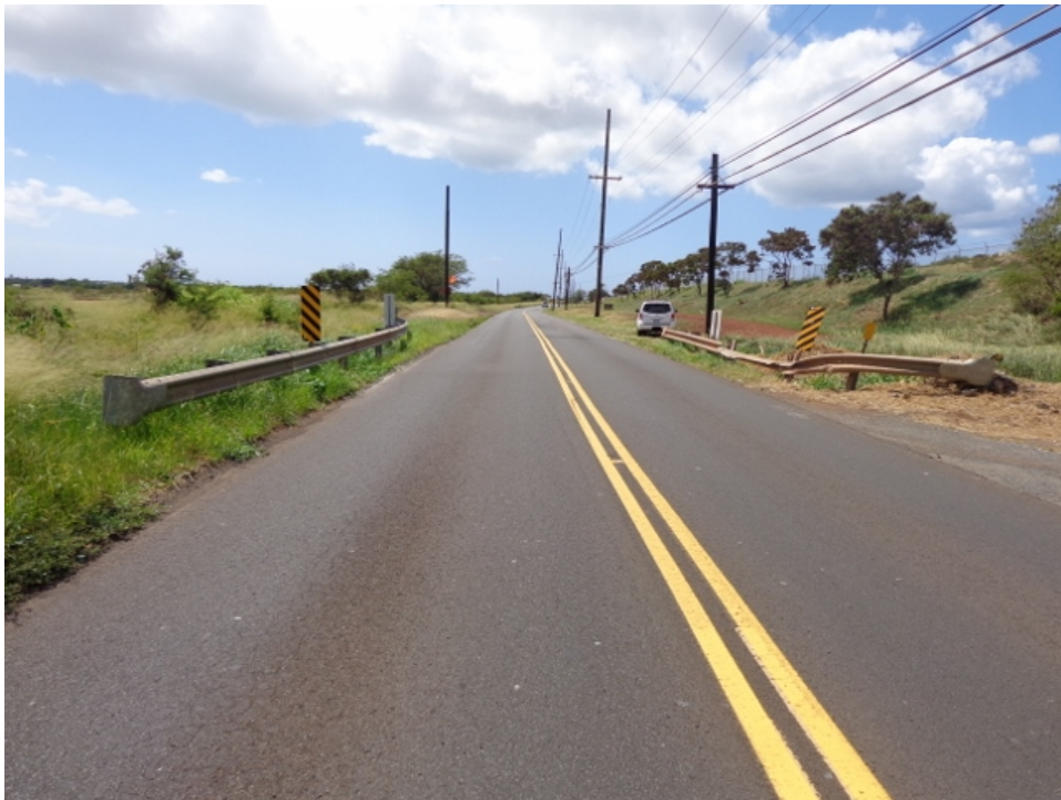
Photo 4: Structure as seen from east approach
