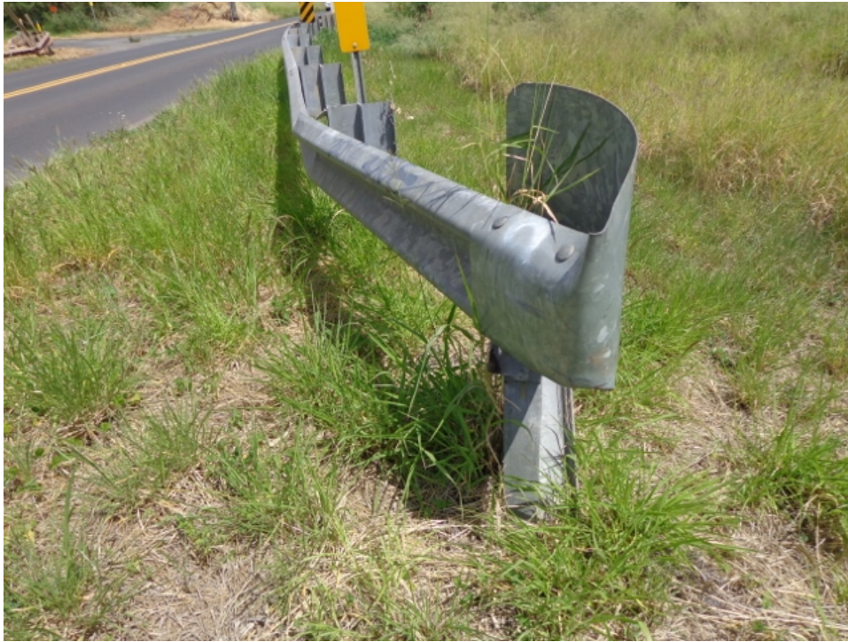
Photo 7: Downstream west approach guardrail end
