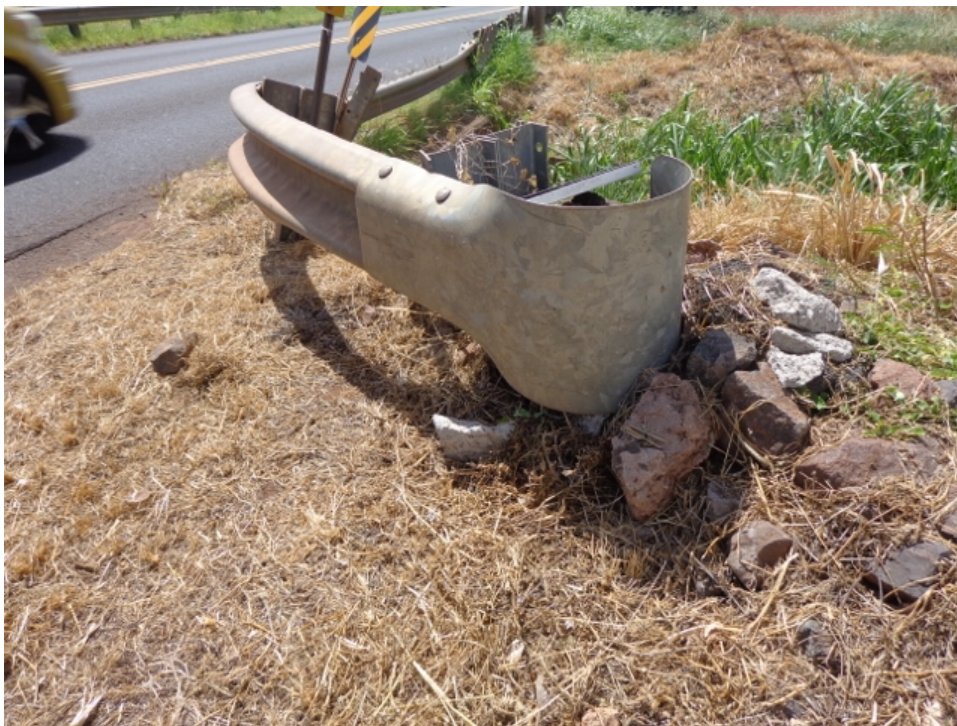
Photo 2: Upstream east approach guardrail end
