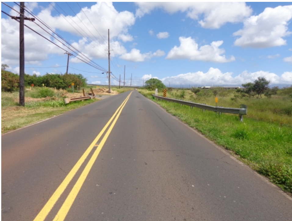
Photo 8: Structure as seen from west approach
