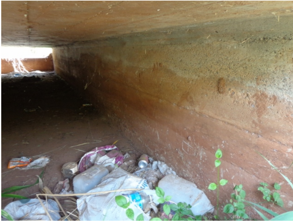
Photo 21: View of west culvert wall
